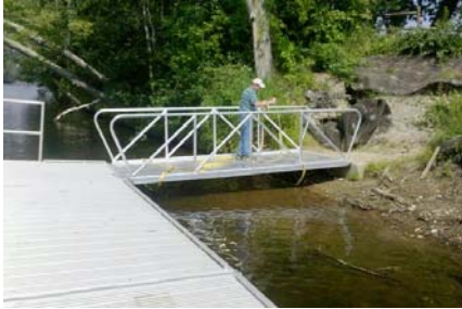
Removal of the harness after installation of the last dock section
